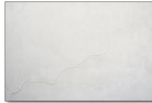
Hairline Cracks
